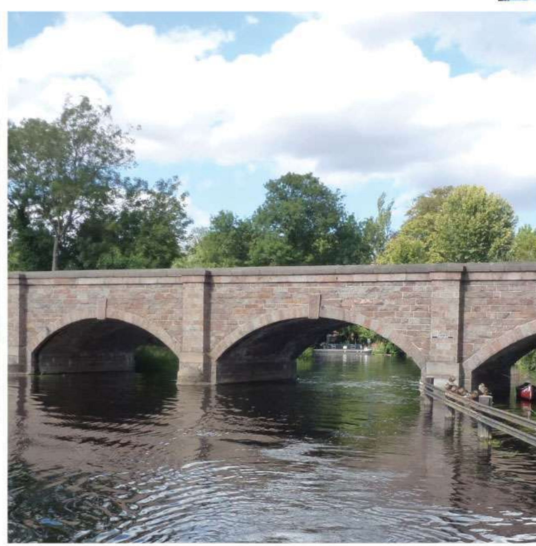
Bridge near point 1
